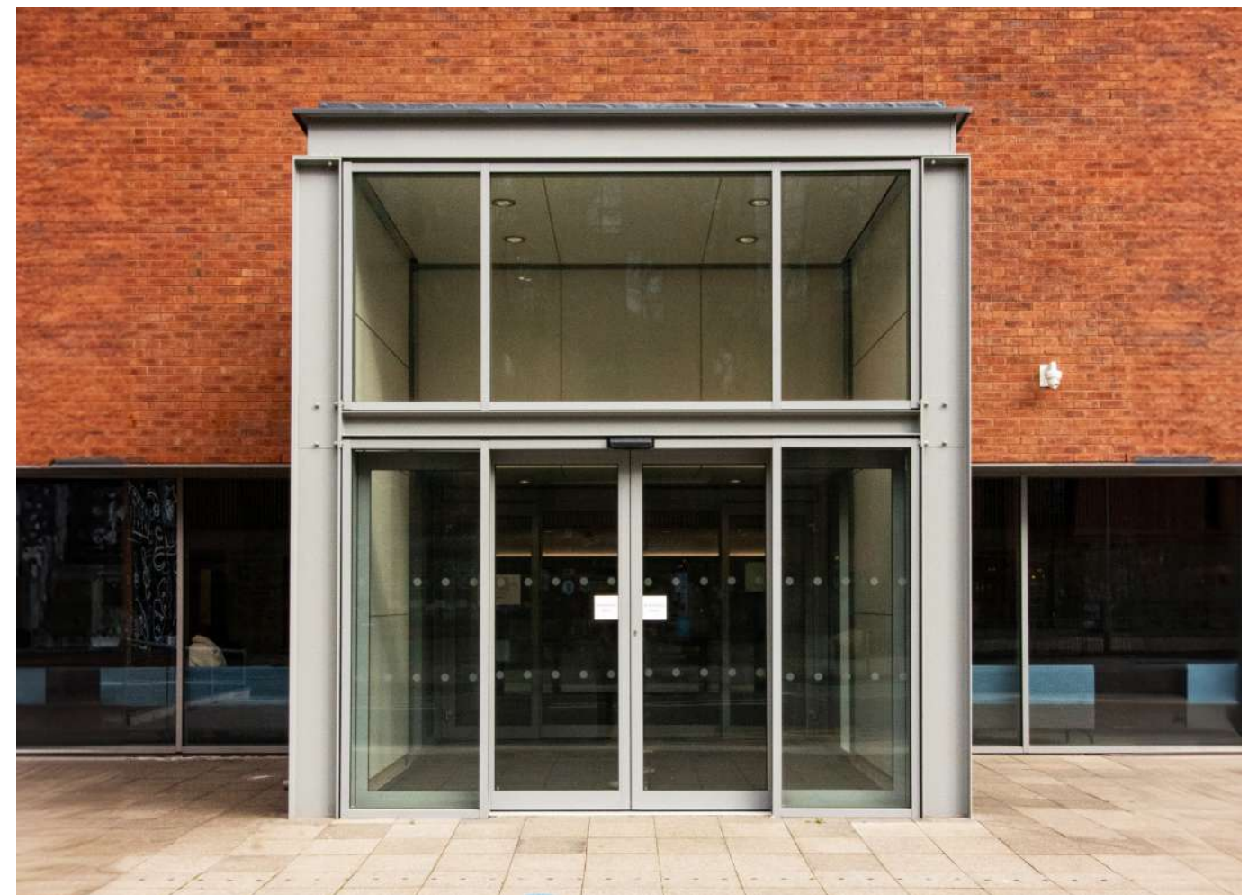
Arts Centre Main Entrance
